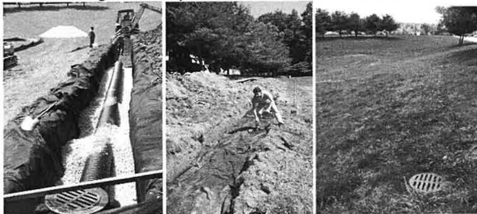
Figure 3: Example of Infiltration Trench Installation
